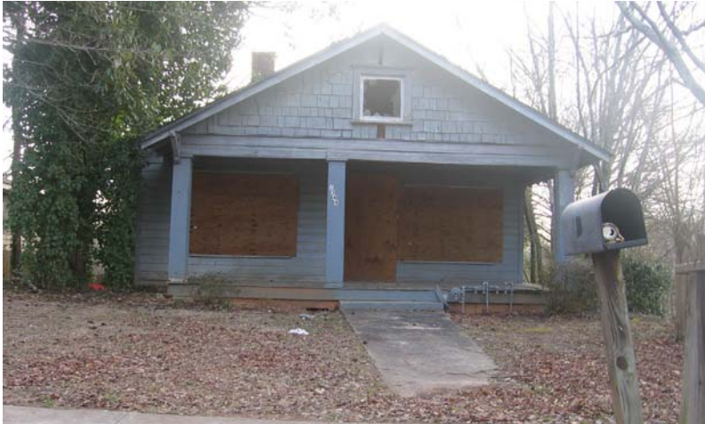
Existing home in need of renovations
