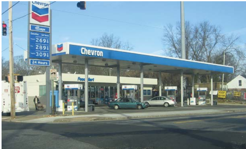
Recently renovated gas station
