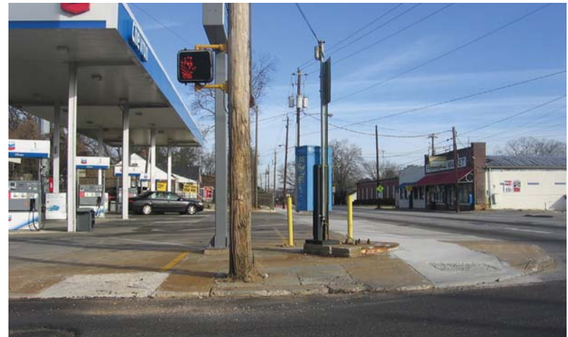
Needed streetscape improvements at pedestrian crossing
